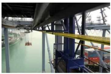
BU: ProfiDAT® data transmission by Conductix-Wampfler is installed in parallel to the existing conductor rails on STS container cranes, or installed in the PE (phase earth) as an integrated configuration. The ProfiDAT® antenna moves inside the profile and is in contact with the transceiver via an Ethernet interface.
